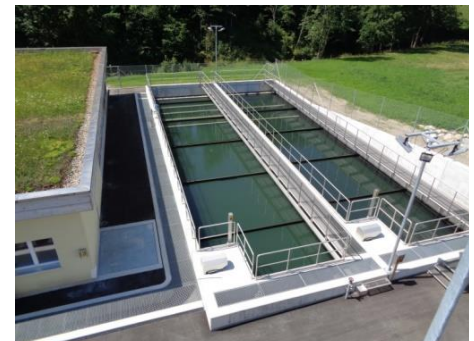
Sedimentationsbecken PAK-Stufe (links Filter)
